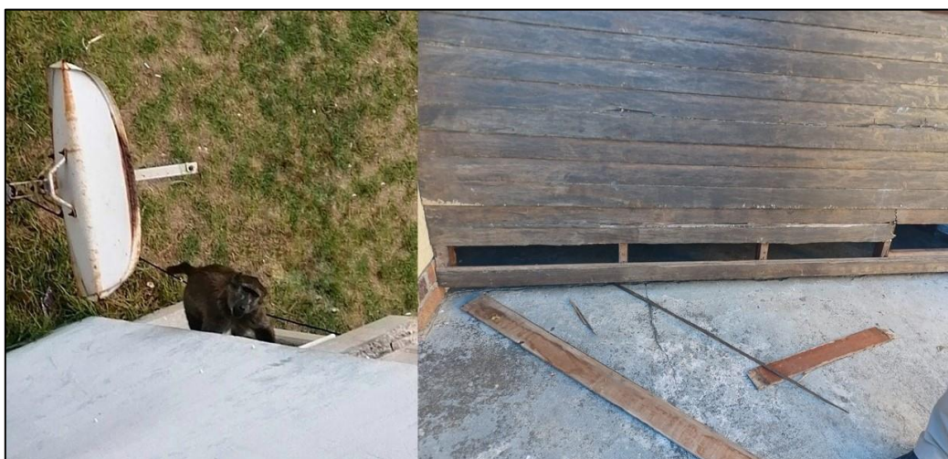
Figure 2. Baboon damage to exterior cabling and garage doors in Da Gama Park. Mitigation advice was provided.
