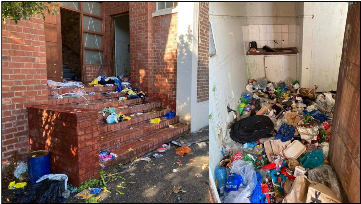
Figure 6. Raided waste room at the ladies' flats in Waterfall Barracks
